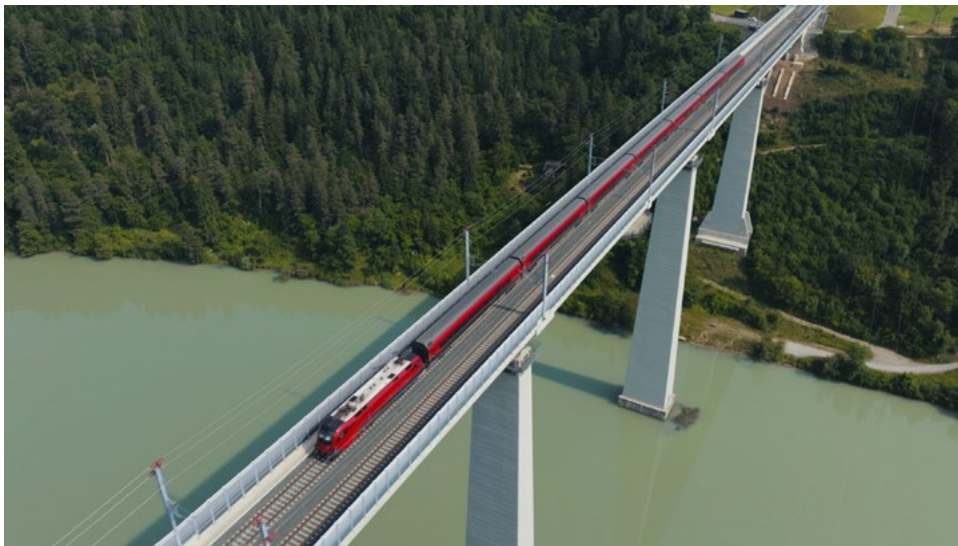
Jauntalbrücke (Bridge over the Jaun Valley), Carinthia © ÖBB
