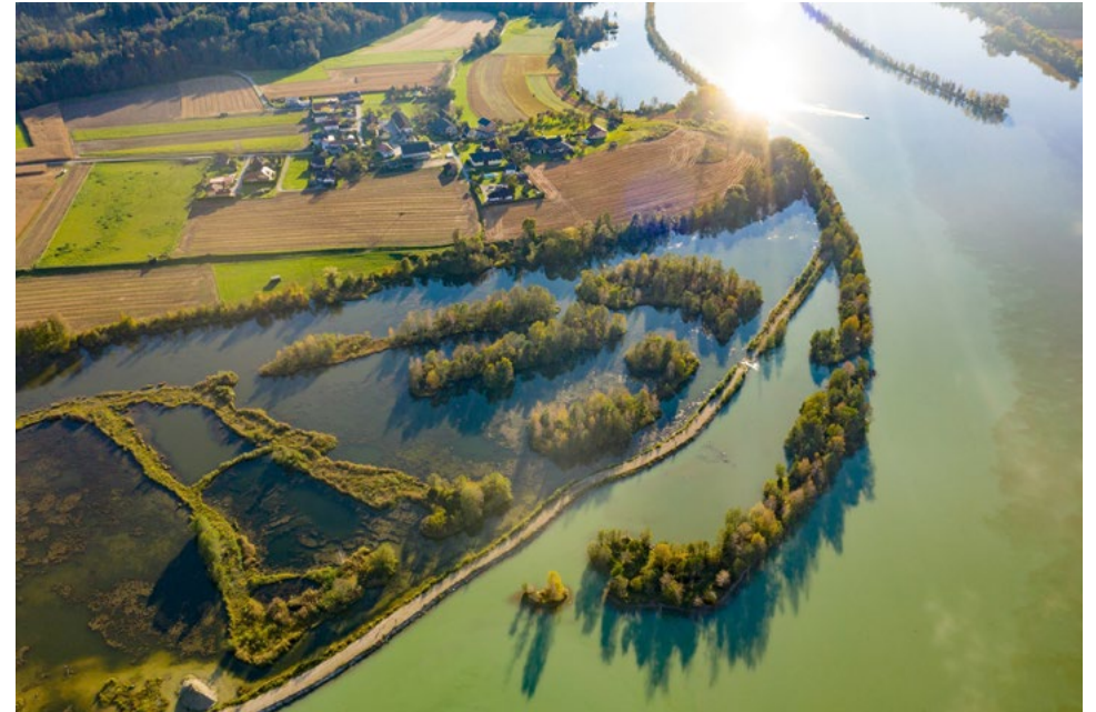
Bird's-eye view of compensatory measures on the Drava River (Völkermarkter reservoir) near Brenndorf, Carinthia © ÖBB/evmedia
